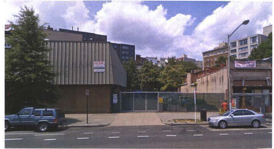
View of existing building on site
