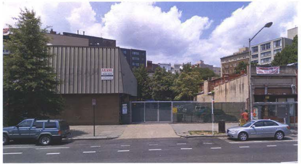
View of existing building on site
