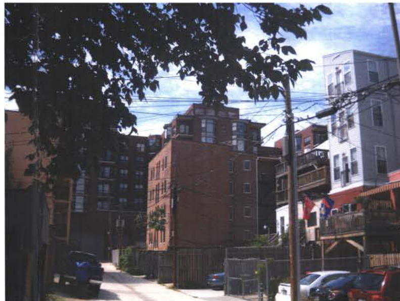
View west from the back alley directly behind the subject property
