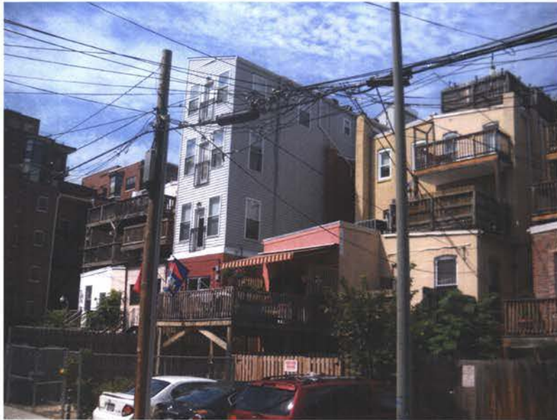
Adjacent properties to the northwest
