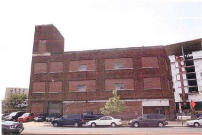
2. North Elevation Along New York Avenue
