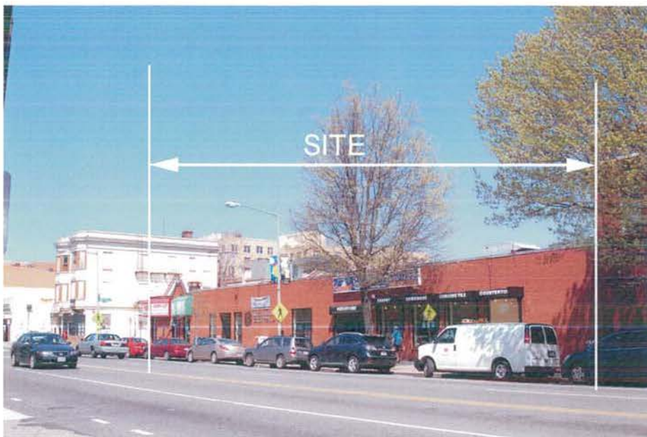
VIEW LOOKING NORTH EAST
