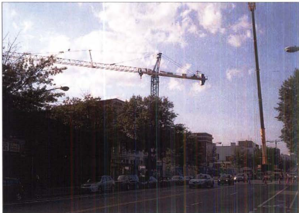
Construction on 14th Street NW
