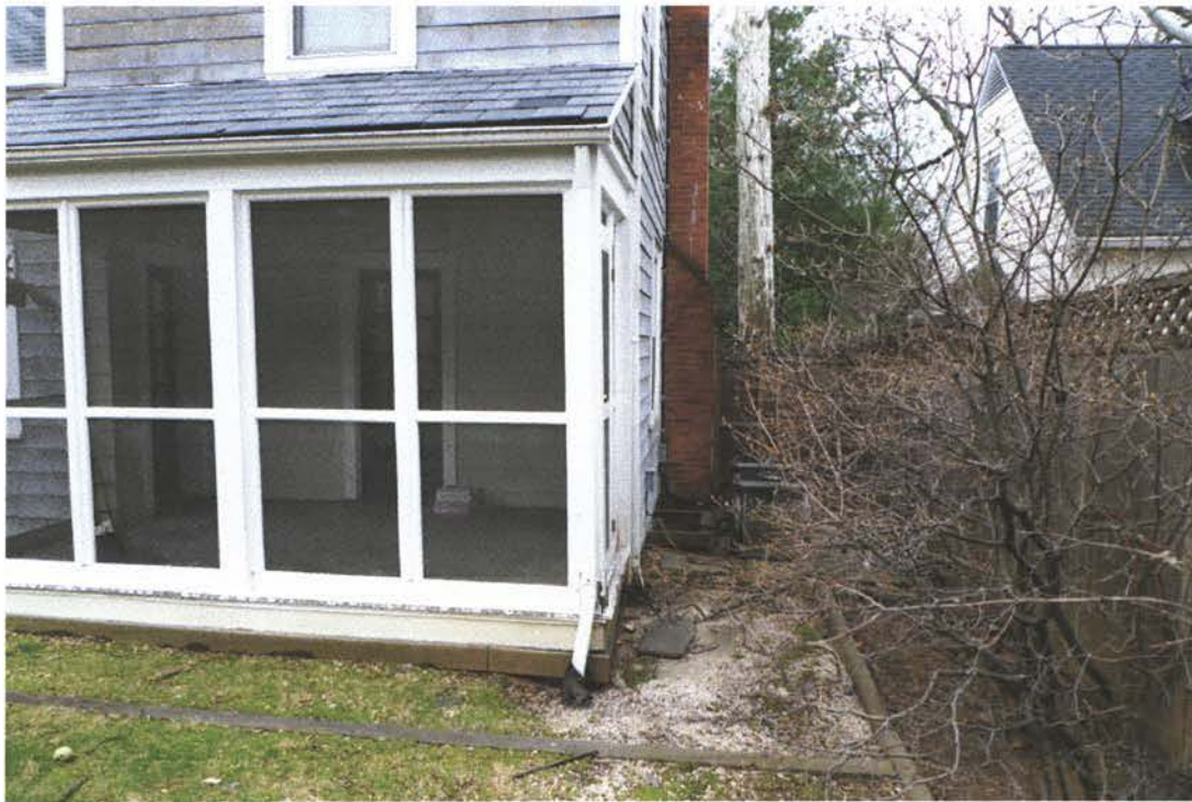
PHOTO 3: REAR OF EXISTING HOUSE AT SCREENED PORCH
