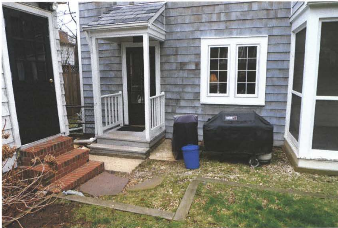
PHOTO 4: REAR OF EXISTING HOUSE AND GARAGE AT REAR DOOR ENTRY
