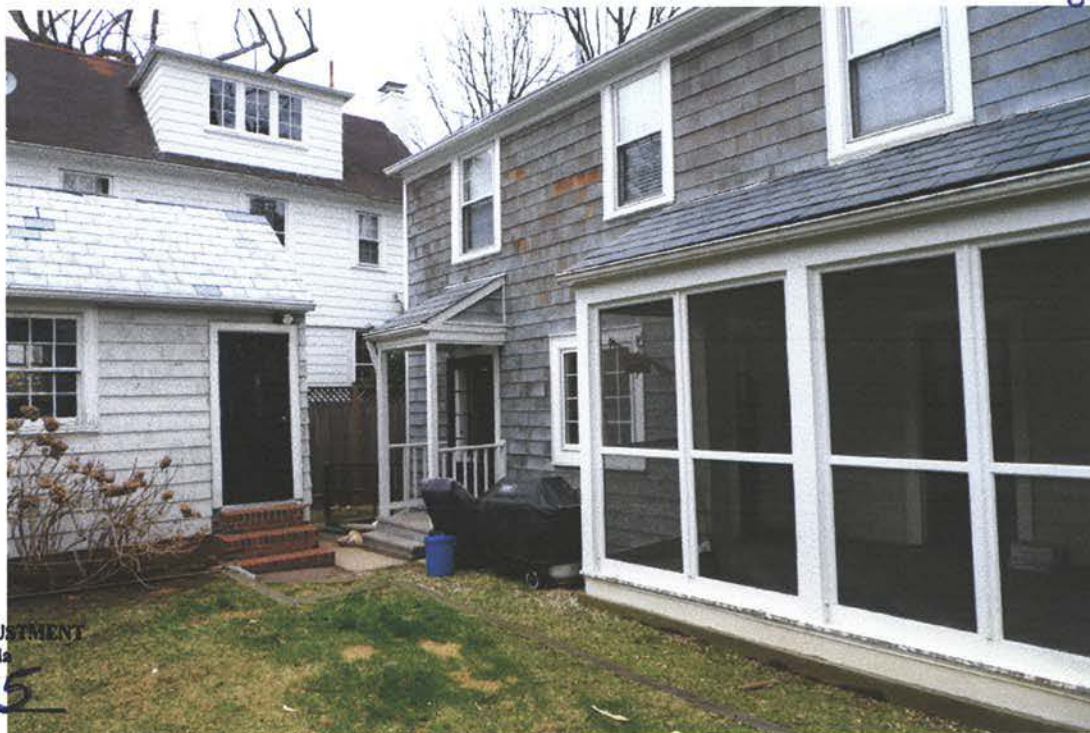
PHOTO 2: REAR OF EXISTING HOUSE AND SIDE OF GARAGE
