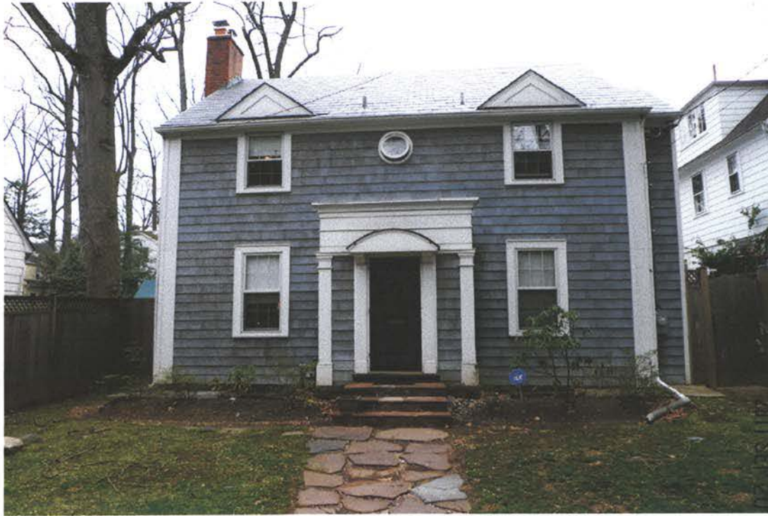
PHOTO 1: FRONT OF EXISTING HOUSE
