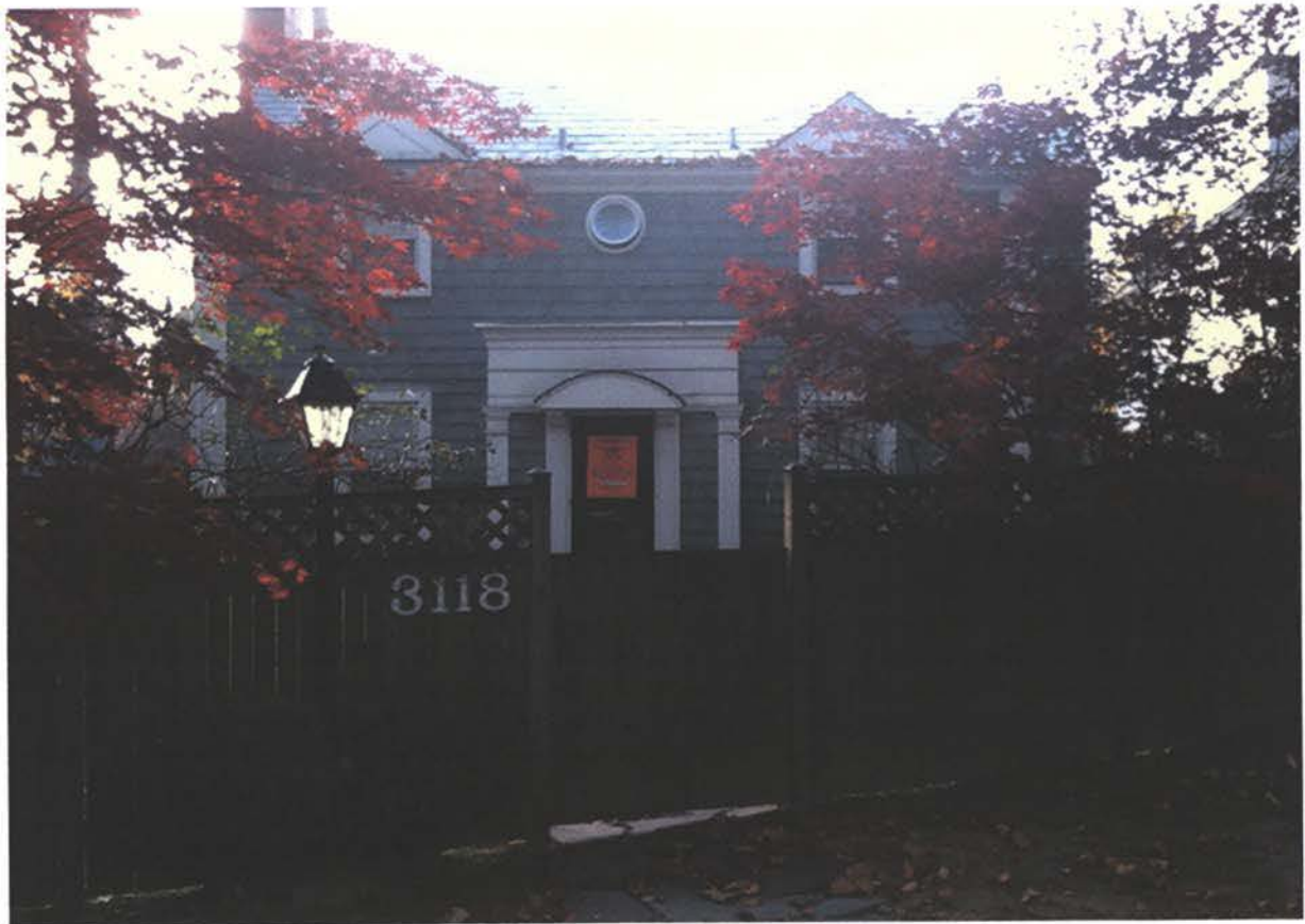
PHOTO 2: FRONT VIEW FROM PUBLIC STREET
