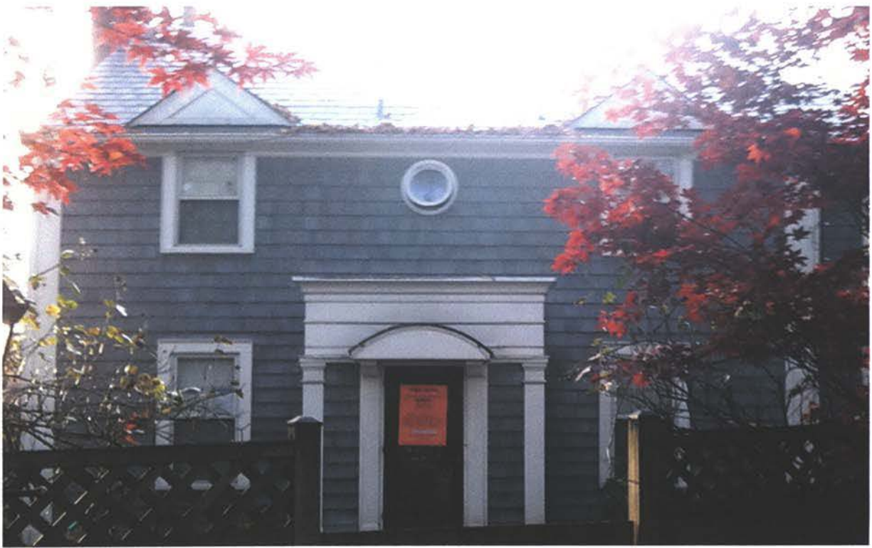
PHOTO 1: FRONT VIEW FROM PUBLIC SIDEWALK
