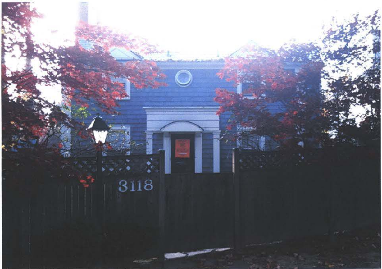
PHOTO 2: FRONT VIEW FROM PUBLIC STREET
