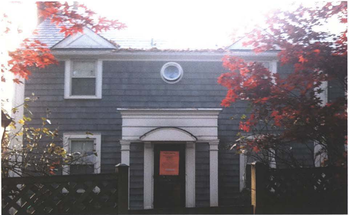
PHOTO 1: FRONT VIEW FROM PUBLIC SIDEWALK
