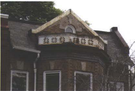
Fig. 11 shows existing cornice to be repaired.
