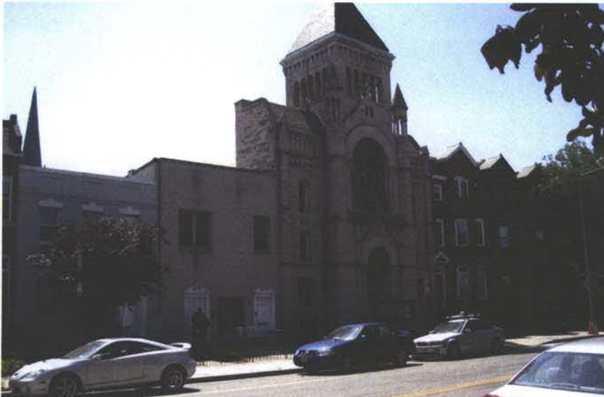
Fig. 10 shows the neighboring apartment house and church.
