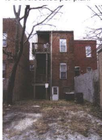
Fig. 14 shows existing rear (east) façade with existing door to basement.
