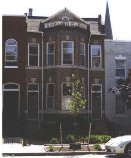
Fig.2. Shows 1633 13 th St.'s original two door configuration.
