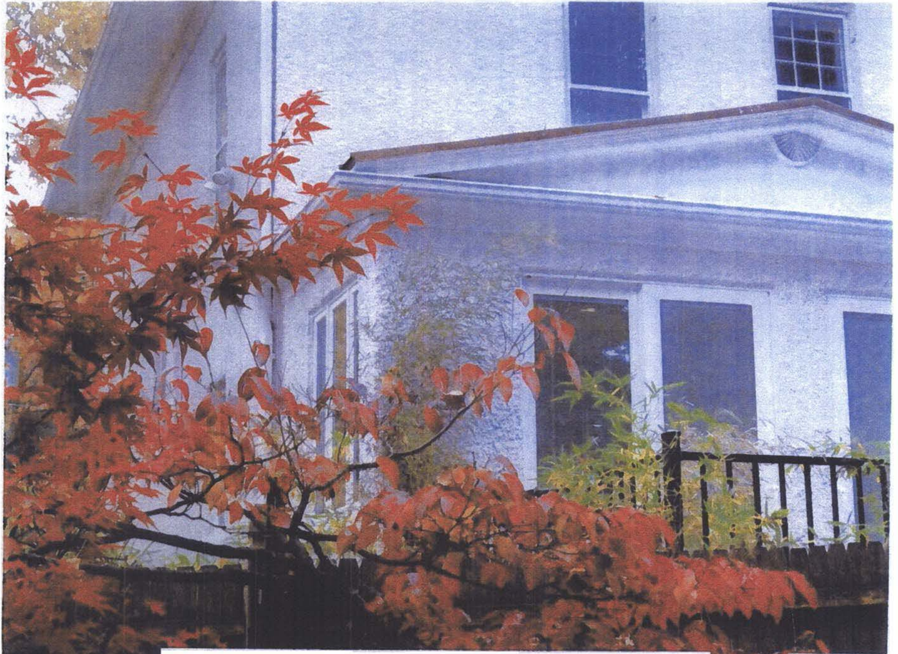
3825 MORRISON NW "AFTER" DECK VIEW C NORTH SIDE
