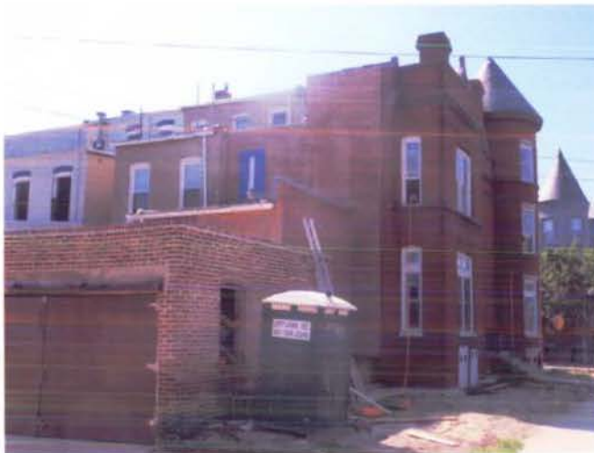
1819 10 th St NW – Existing alley view
