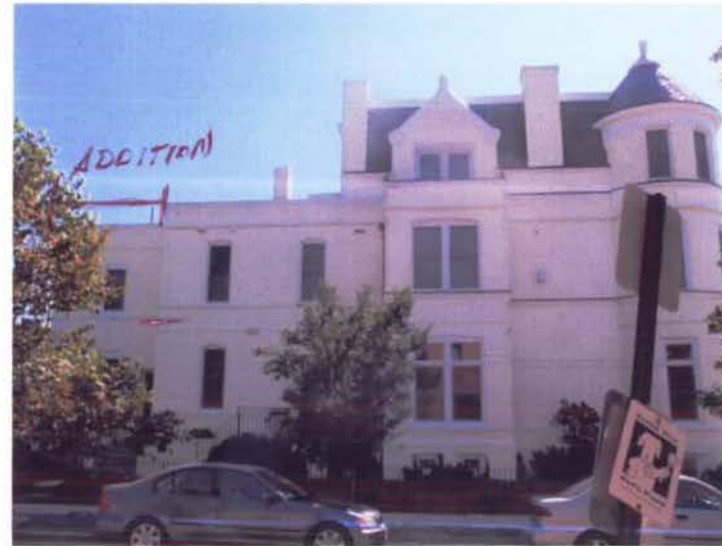
1801 10 th St NW – existing addition as requesting
