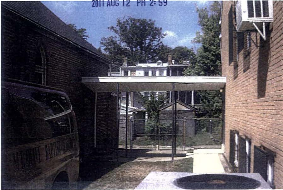
Current Breezeway Between the Old and New Church
