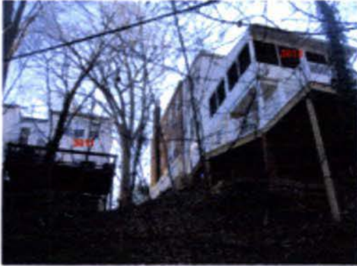
NEIGHBORING HOUSE LOCATION - VIEWS FROM ALLEY
