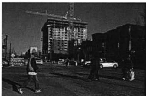
Construction cranes line K Street, one of the areas where several apartment complexes are being built. Lexey Swall for The Wall Street Journal
