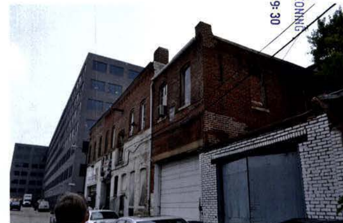
BACK ALLEY - LOOKING SOUTH EAST
