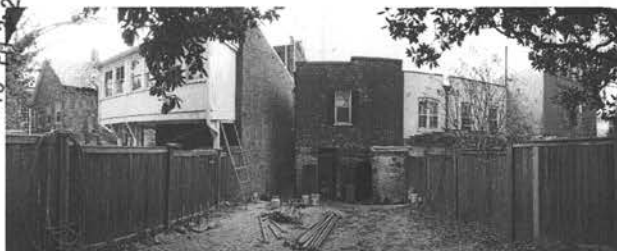
2 REAR YARD LOOKING SOUTH CFA.02
