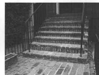
8 EXTERIOR STAIR @ 3127 P STREET NW CFA.02
