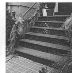
9 EXTERIOR STAIR @ 3129 P STREET NW CFA.02
