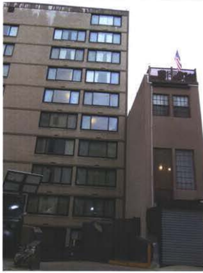
ALLEY (10' WIDE) ALONG REAR OF PROJECT SITE
