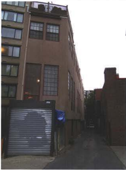
ADJACENT BUILDINGS IN LOCATED IN REAR OF PROJECT SITE
