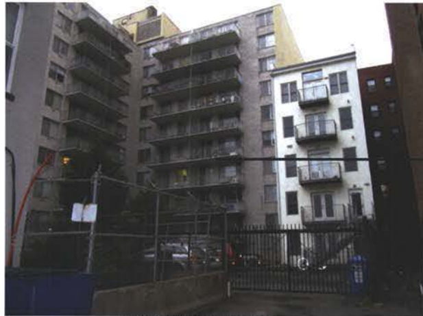
VIEW OF EXISTING ADJACENT BUILDINGS FROM REAR ALLEY
