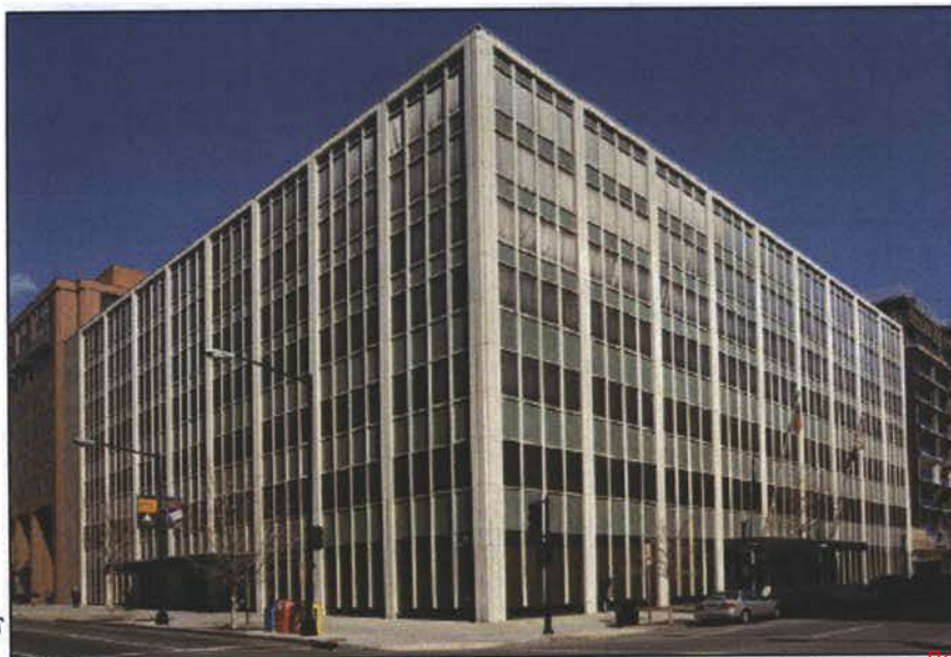
2055 L Street, NW: View from southwest
