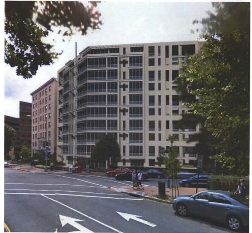
VIEW LOOKING ACROSS NEW HAMPSHIRE AVENUE NW
