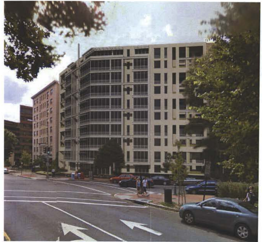
VIEW LOOKING ACROSS NEW HAMPSHIRE AVENUE NW
