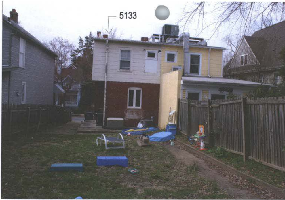
view of rear
