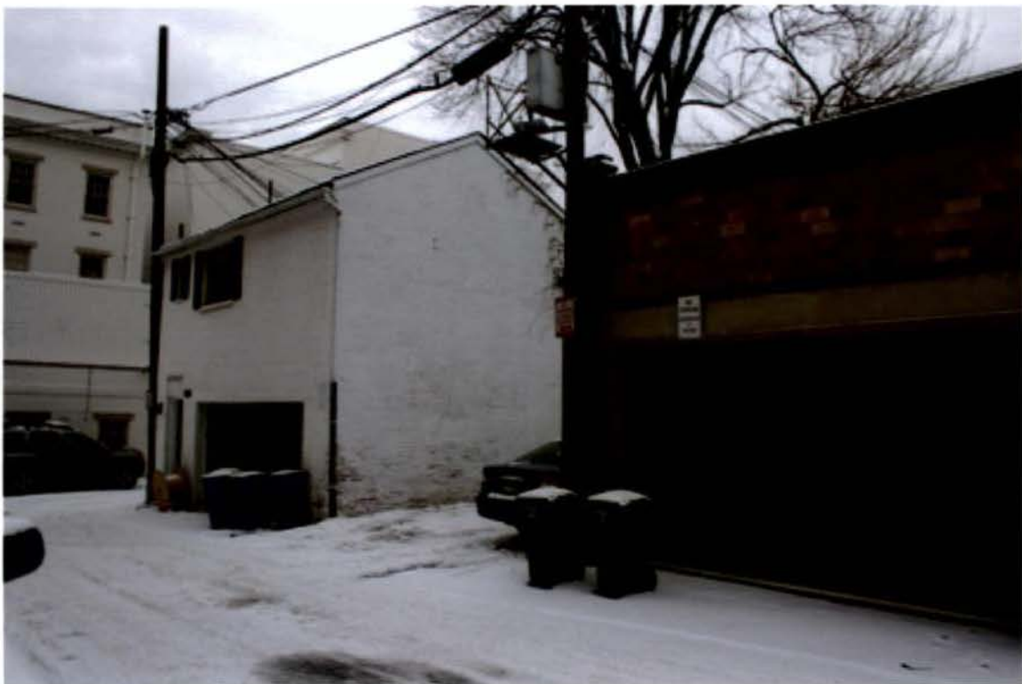
ALLEY VIEW TO WEST
