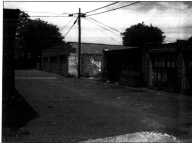
④ View from Alley Looking West
