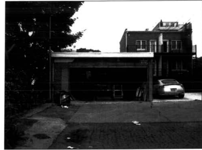
① Garage Elevation from Alley
