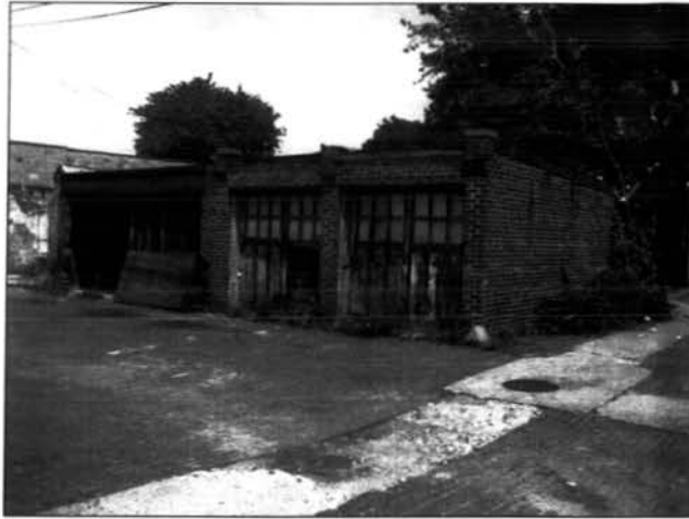
③ View from Alley Looking North at Adjacent Garage
