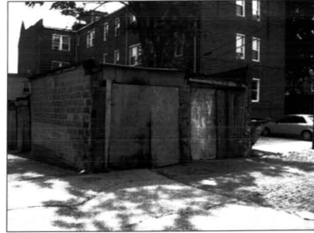
① View from Garage Looking East
