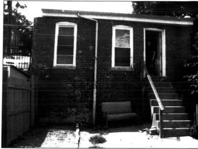
③ Garage Elevation from Backyard
