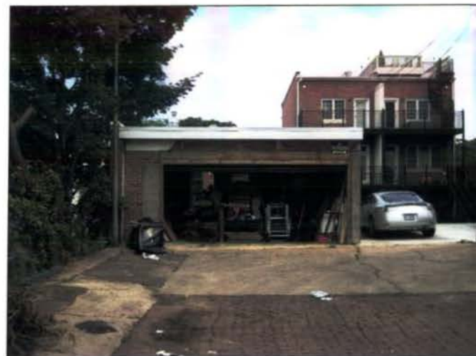
① Garage Elevation from Alley
