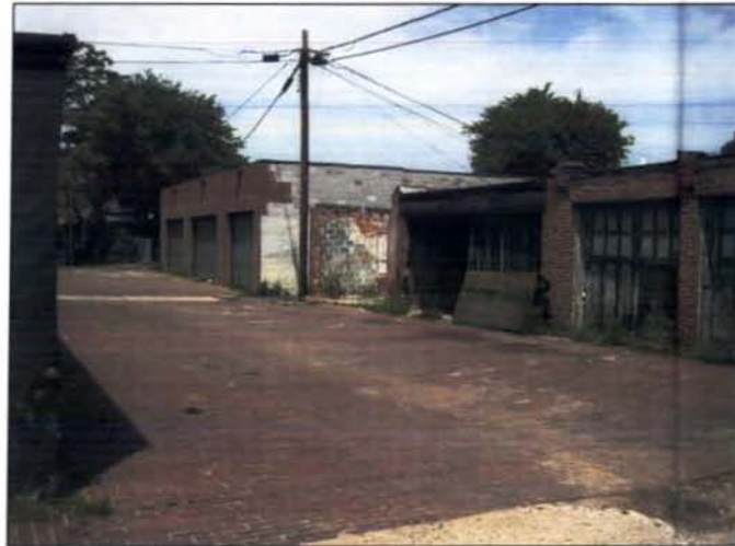
④ View from Alley Looking West
