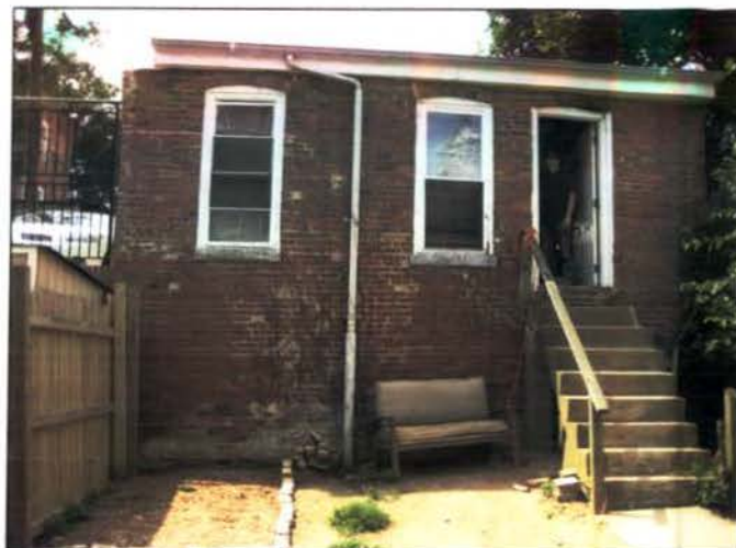
③ Garage Elevation from Backyard
