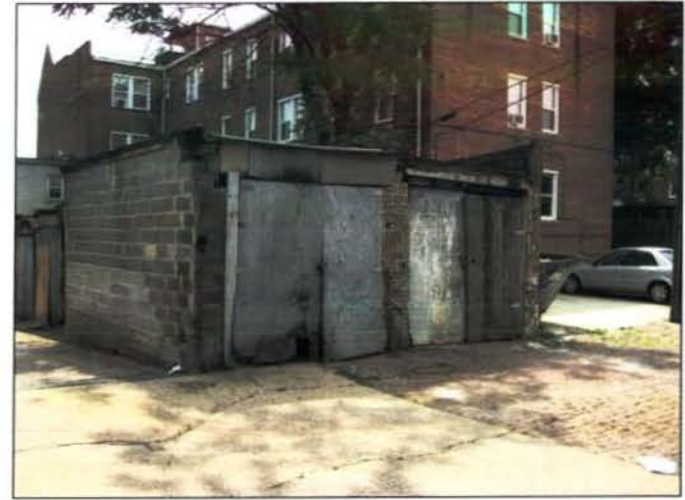
① View from Garage Looking East
