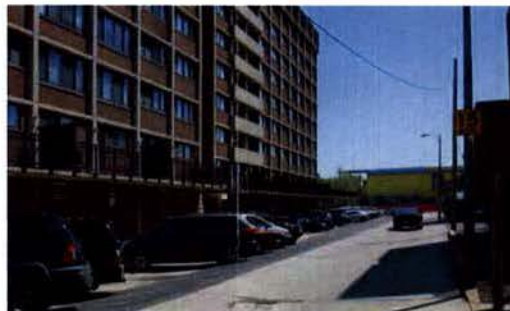
8. VIEW OF PUBLIC ALLEY LOOKING SOUTH
