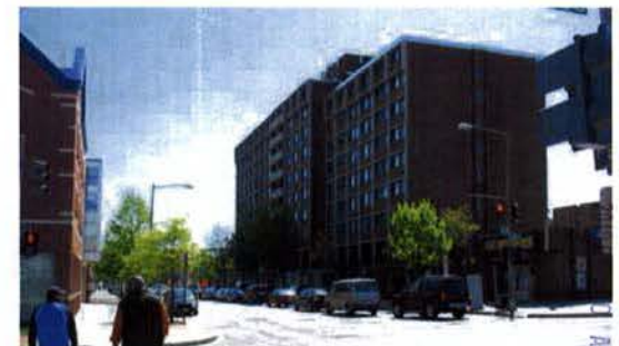
9. VIEW FROM S STREET LOOKING SOUTH
