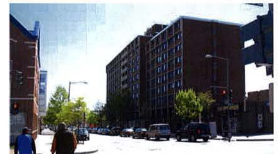
9. VIEW FROM S STREET LOOKING SOUTH
