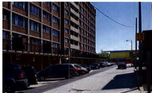
8. VIEW OF PUBLIC ALLEY LOOKING SOUTH
