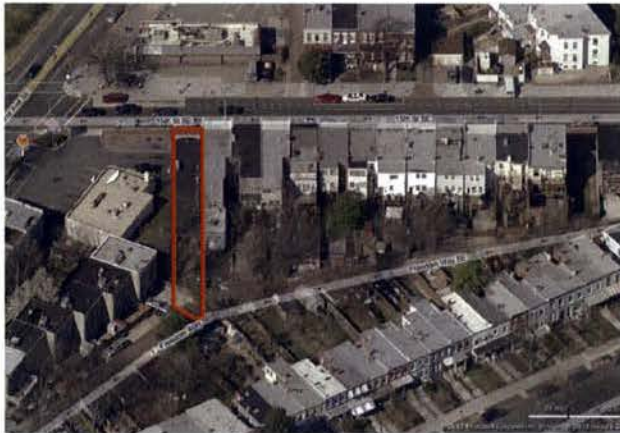
VIEW FROM FREEDOM WAY, LOOKING WEST
