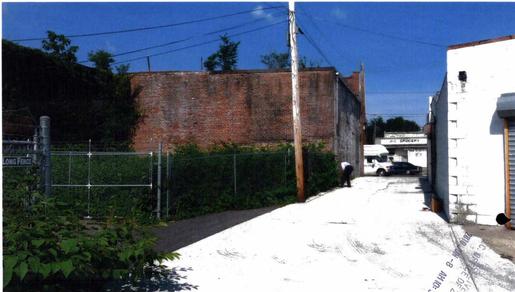
Photo 4 - Strand Treater (rear elevation) looking east along public alley
