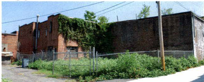
View of rear of lots from public alley
