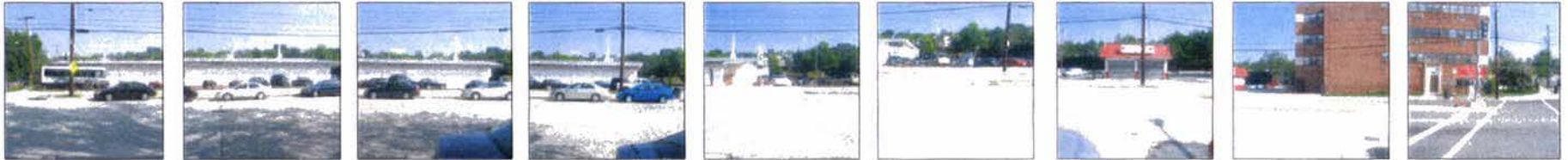
SEGMENT WEST OF DIVISION AVE NE
