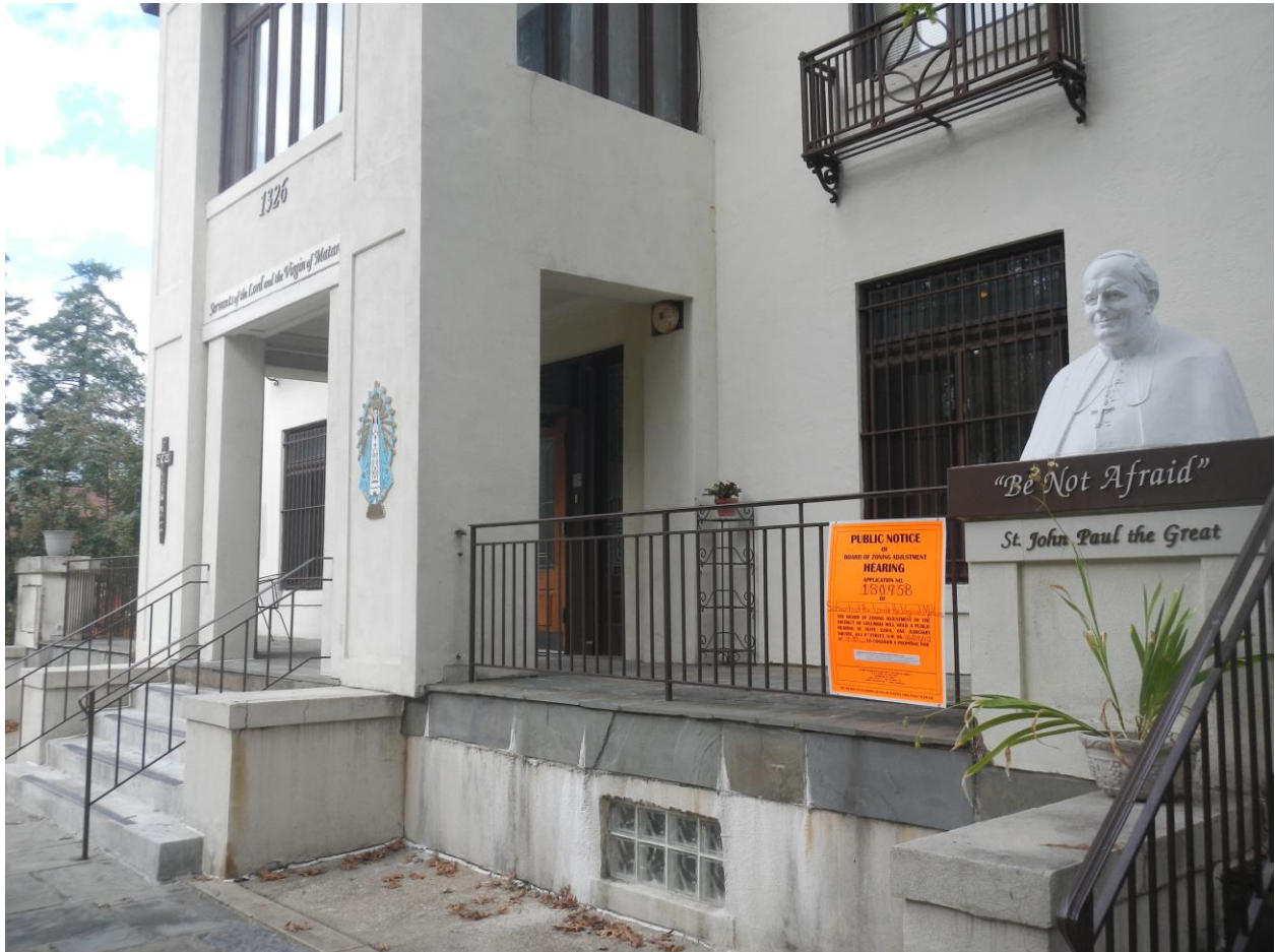
Photo-3-18095B FORM 145 Servants of the Lord and the Virgin of Matará 1326 Quincy Street NE on building (detail up-close)
