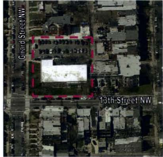
View of the site looking west
