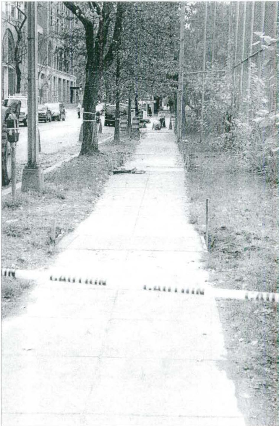
DDOT Sidewalk Repairs and Replacement
