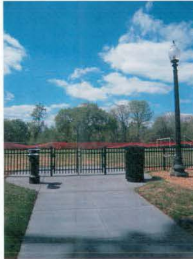
Photo 5: Francis Field – Secondary Entrance with water fountain, trash receptacle, and park light.
