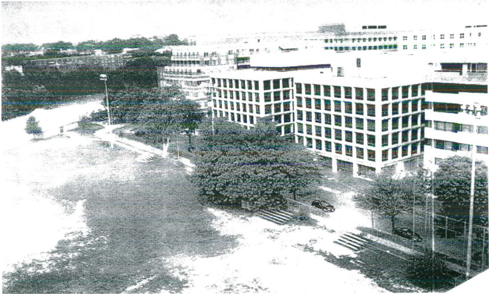
Francis Field and BNA Buildings, 2006
