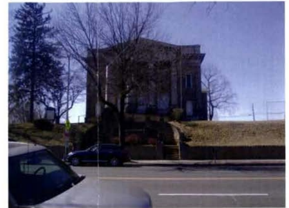
VIEW FROM GEORGIA AVE LOOKING W
