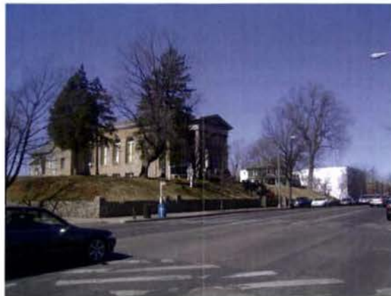
VIEW FROM GEORGIA AVE LOOKING NW
