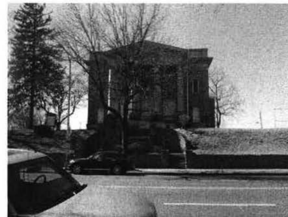
VIEW FROM GEORGIA AVE LOOKING W
