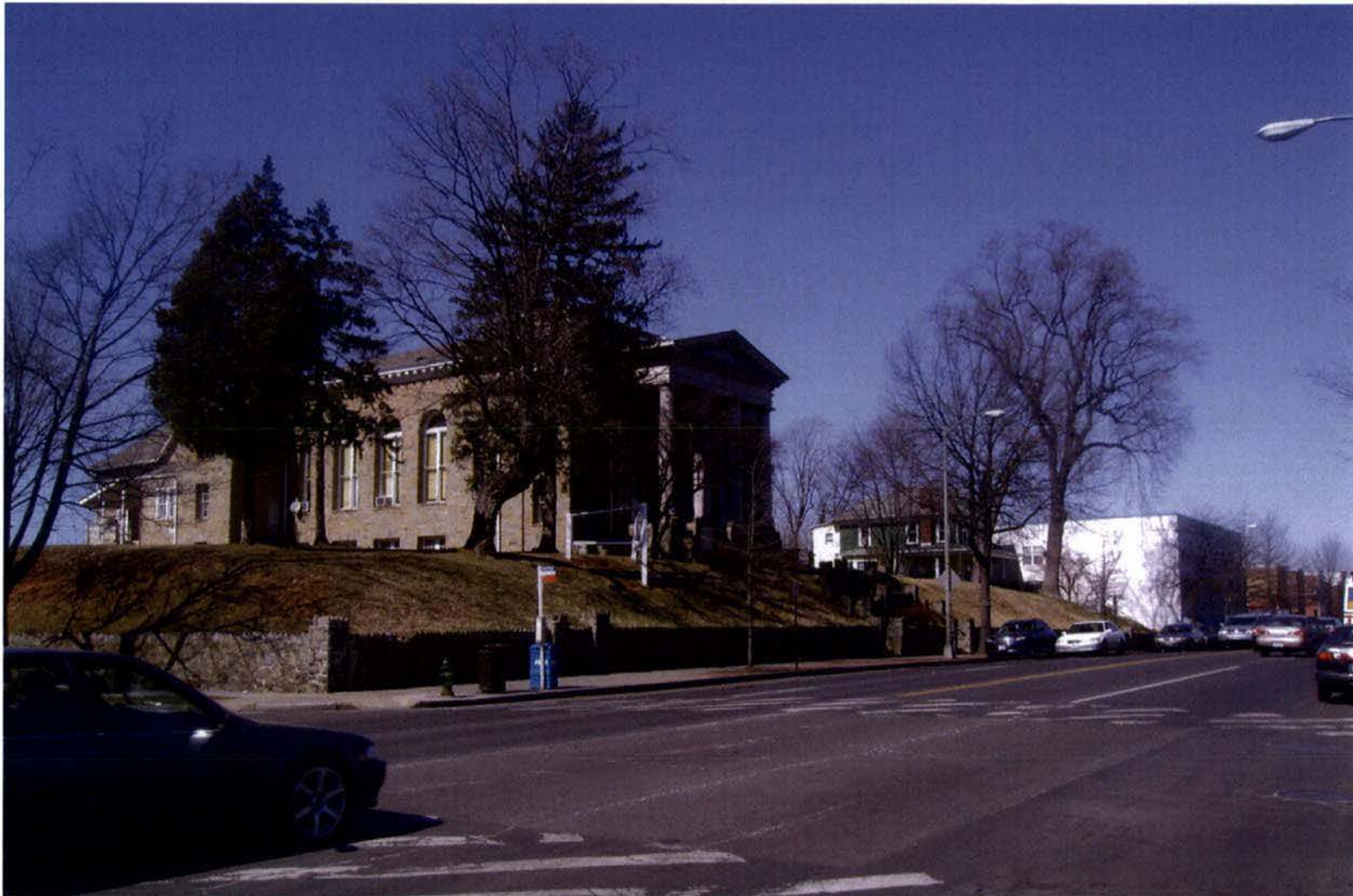
VIEW FROM GEORGIA AVE LOOKING NW
