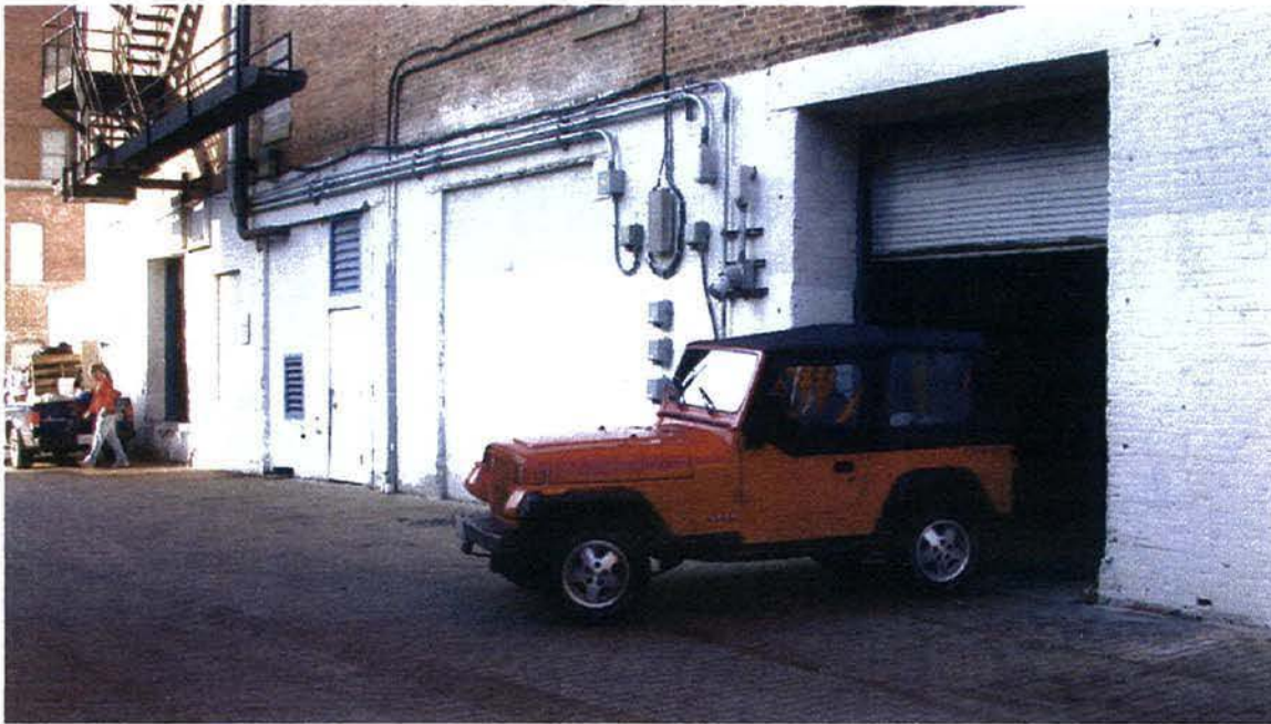
PALOMA WAY, REAR OF EXTRA SPACE STORAGE W/DRIVE THROUGH FROM INTERIOR OF BUILDING
