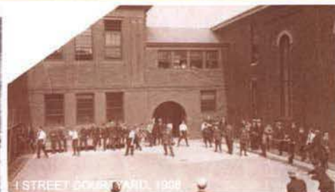
1 STREET COURT YARD, 1908
