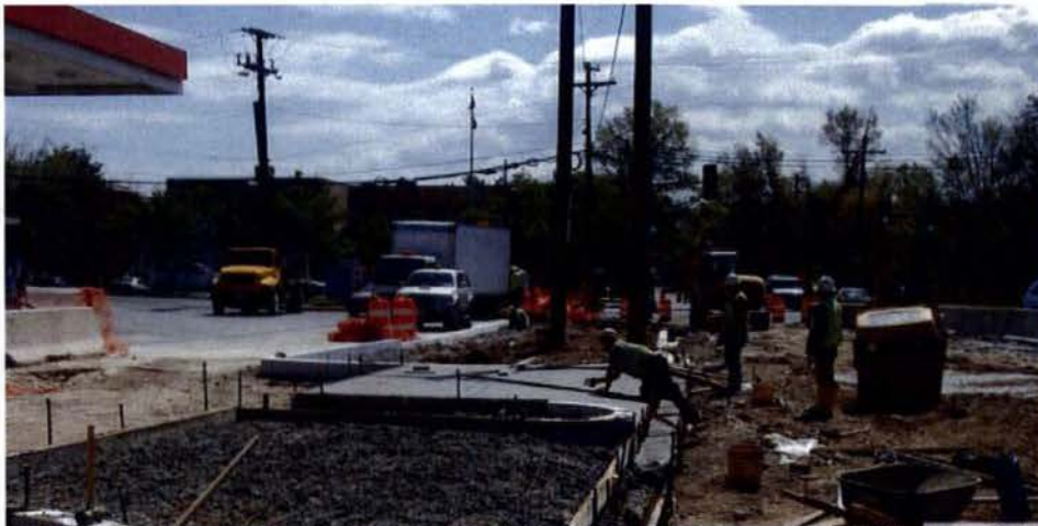
New sidewalk in front of Exxon on South Dakota Avenue NE
