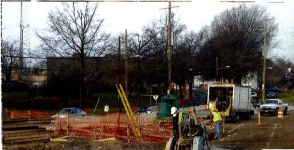
Brickwork for the construction channel on South Dakota Ave NE
