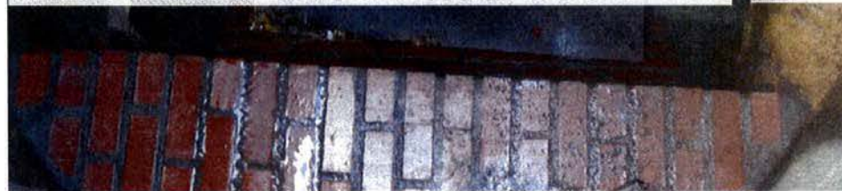
Construction brick channel inside manhole on South Dakota Ave NE
