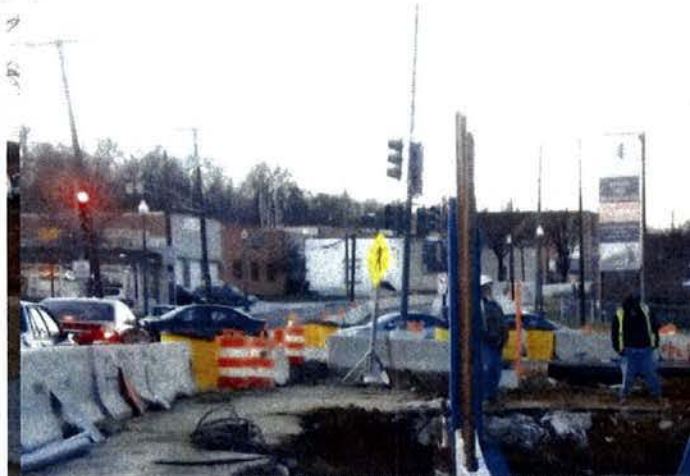
New sidewalk on Riggs Road and South Dakota Ave NE
