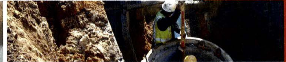
Installation of sewer manhole on South Dakota Ave NE
