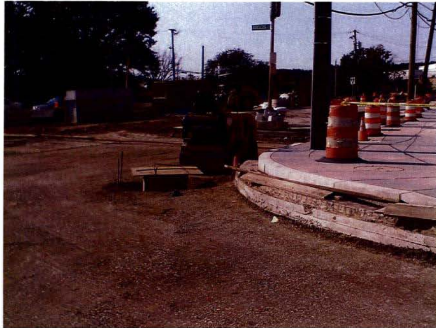
Compaction and grading work of the graded aggregate base in the preparation for the installation of the roadway at the north west corner of Riggs Road and 3 rd St.
