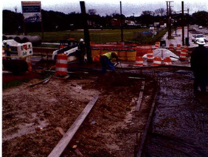
Formwork preparation for the placement of concrete for the installation of the sidewalk on Riggs Road; at 3 rd Street north west corner
