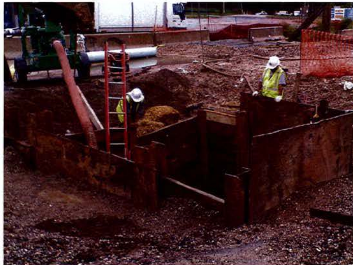
Continued shoring and dewatering work at the location of manhole M36 on South Dakota Ave north of Kennedy Street
