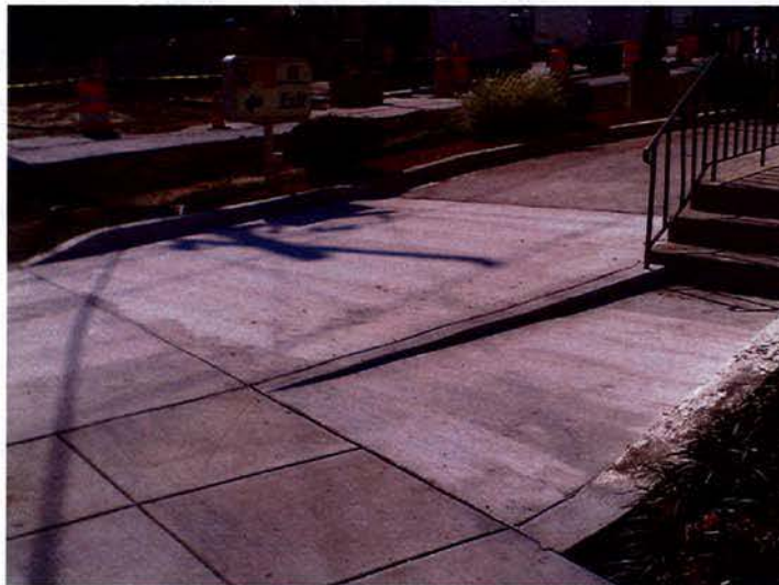
Newly installed driveway on 3 rd Street; west side north of Riggs Road, for the Taco Bell property.
