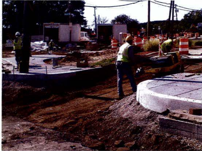
Grading and compaction work for the installation of the driveway on 3 rd Street; west side north of Riggs Road.
