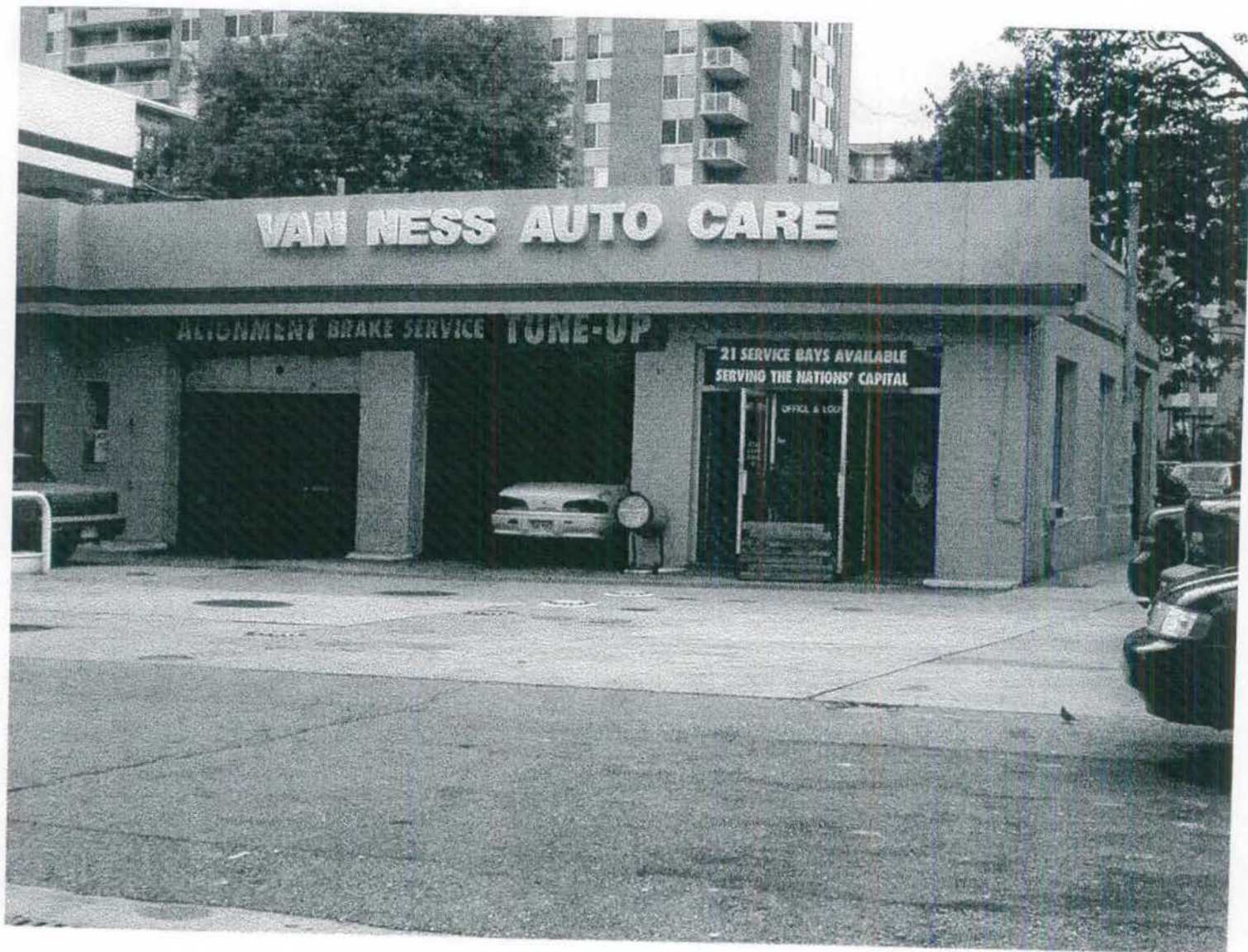
Front of 4225 Connecticut Avenue showing office and Van Ness South
