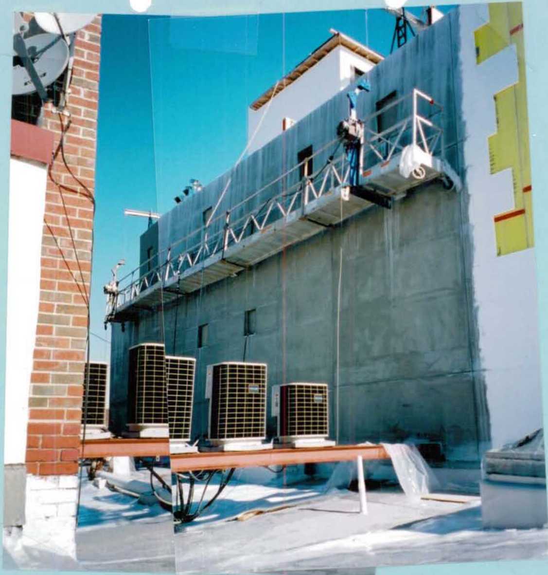
VIEW FROM 1823 BELMONT ROAD, NW, "B" LOOKING NORTHEAST
