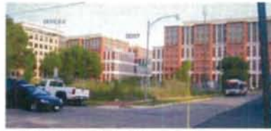
2. VIEW SOUTHEAST TOWARDS DEPARTMENT OF TRANSPORTATION
