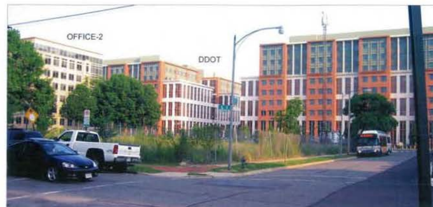
2. VIEW SOUTHEAST TOWARDS DEPARTMENT OF TRANSPORTATION
