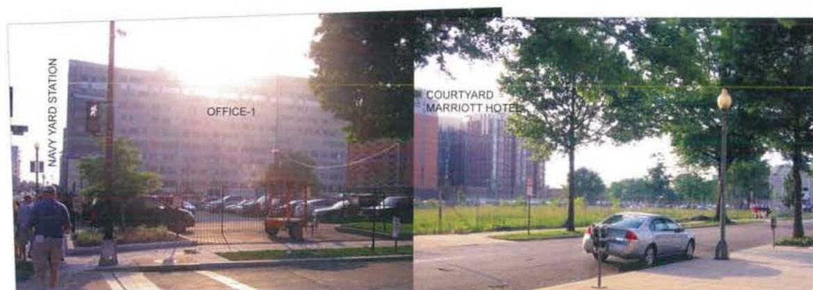
3. VIEW NORTHWEST TOWARDS COURTYARD MARRIOTT HOTEL
