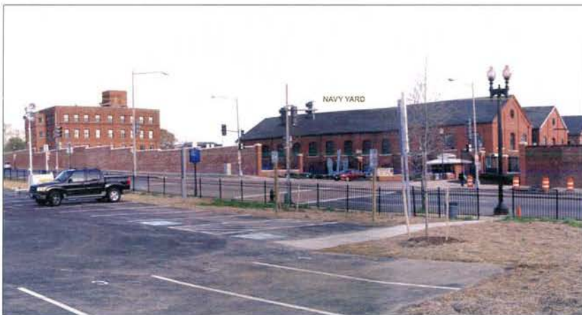
3. VIEW SE TOWARDS NAVY YARD
