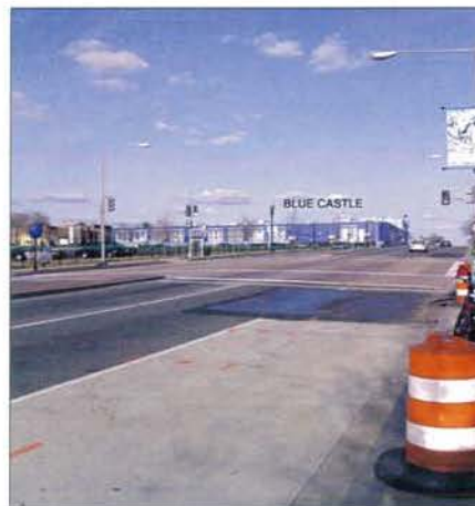
4. VIEW EAST ALONG M STREET SE
