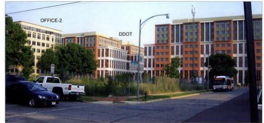
2. VIEW SOUTHEAST TOWARDS DEPARTMENT OF TRANSPORTATION
