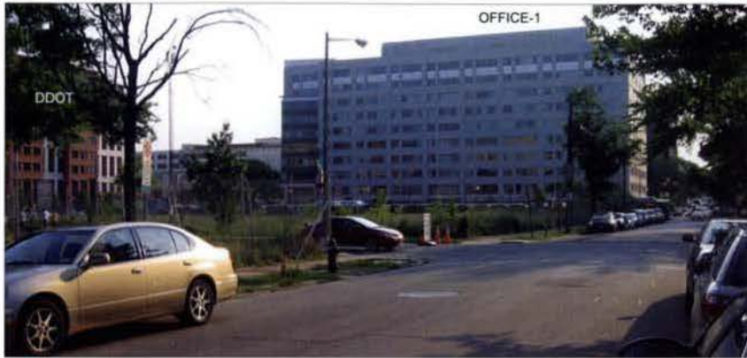
1. VIEW WEST ALONG L STREET SE
