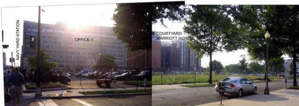
3. VIEW NORTHWEST TOWARDS COURTYARD MARRIOTT HOTEL
