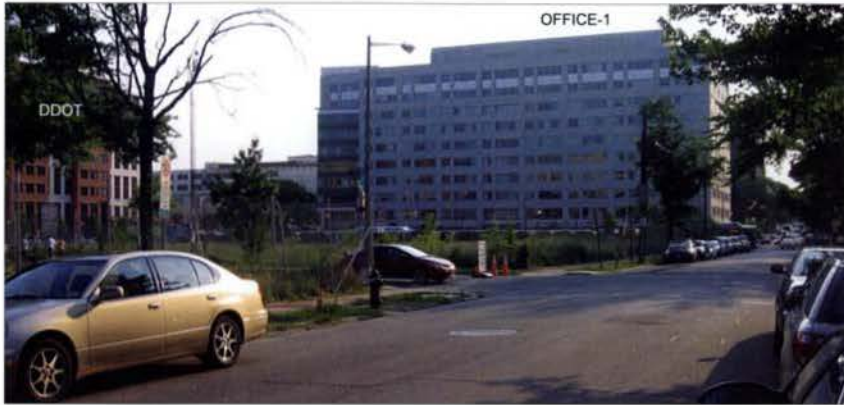
1. VIEW WEST ALONG L STREET SE
